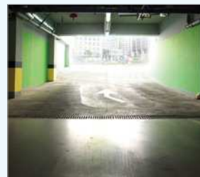
Indoor Parking Entrance
